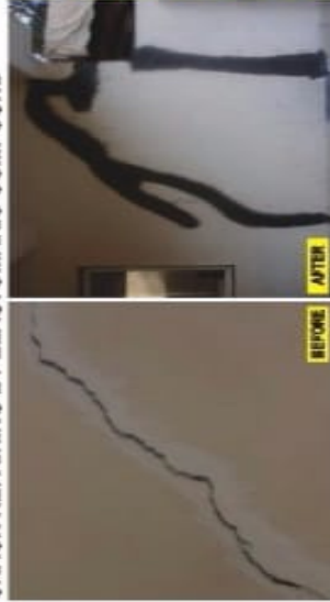
CRACK REPAIRING BY ELASTOMERIC COMPOUND
